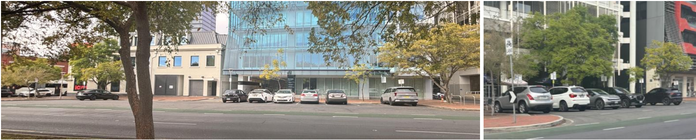
Figure 4-18: Light Square/Wauwi – Eastern Side Parking Conditions
